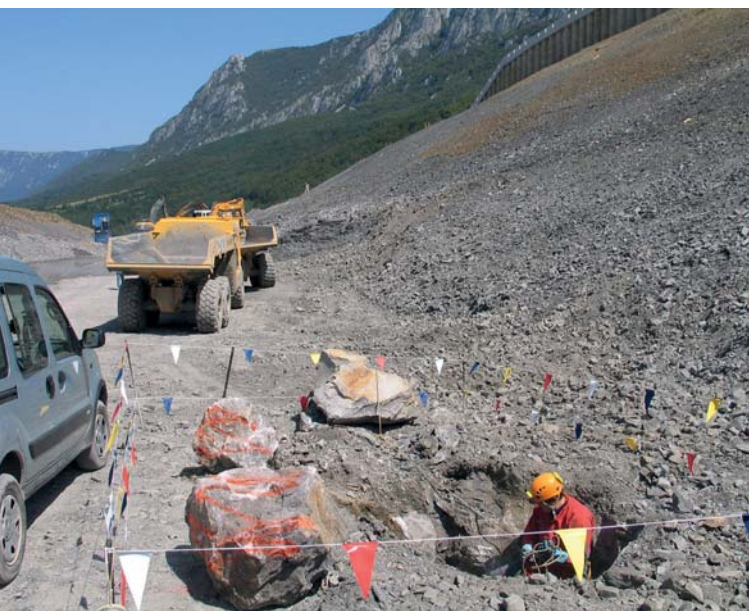
13 Vhod v jamo v flišu. The entrance to a flysch cave.
