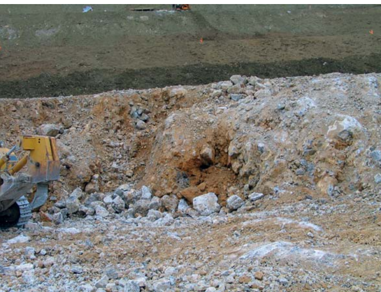
11 Jama, zapolnjena z naplavino. A cave filled with sediment.
