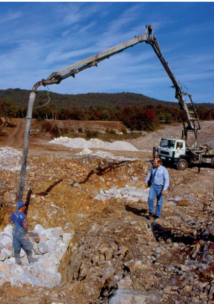
4 Zapiranje špranjaste jame. Closing up a fissured cave.
