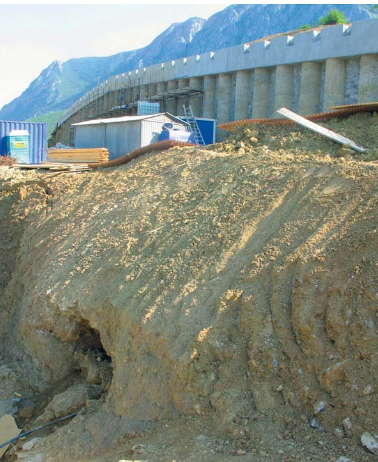
10 Jama z vodnim tokom na stiku breče in fliša. A cave with the water flow at the contact of breccia and flysch.
