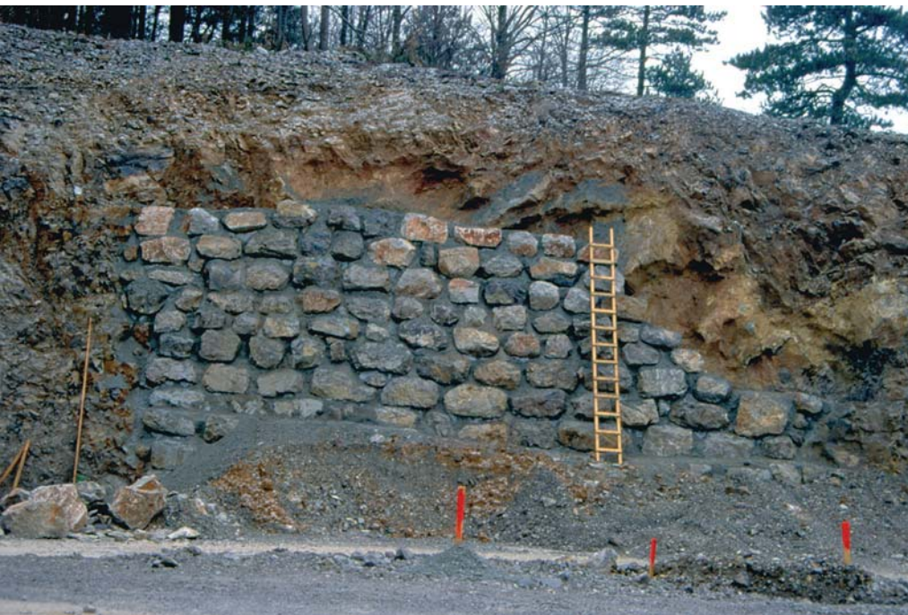
12 Zapiranje jame v brežini useka. Closing a cave in the slope of the cut.
