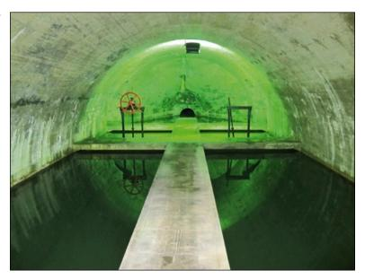
The so-called "Military Water Supply System" was built simultaneously with the public, civil water supply system. It lifted water from the Sv. Ivan spring by means of two piston pumps by as much as 950 m (which due to exceptionally high pressures is rare even nowadays) to the Žbevnica reservoir, and than utilised gravity to supply the then border area all the way from Hrpelje – Kozina to Klana and Mučići.
