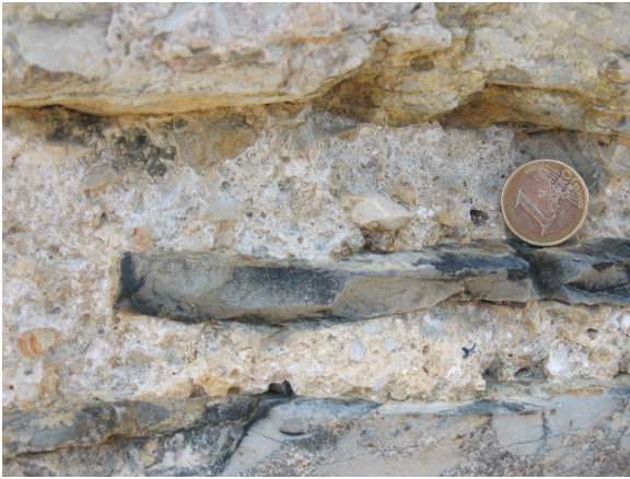
Fig. 9.3: The mortar used in the construction of the tower was made from dolomite chippings, sand and lime. Chippings measure up to 2 cm. View 1.
