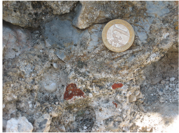
Fig. 9.13: Mortar in the inner curtain wall. The mortar was made from lime and gravelly sand from the Sava river. Brick fragments were found within the mortar. View 2.
