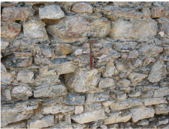
Fig. 9.5: The tower wall. Almost exclusively, quarry stones from the top of the Smlednik Castle Hill were used. The quarry stones in tower walls were coarse and heterogeneous – they came in different shapes and sizes. As a rule their edges were not chiselled. The construction was not rough.
