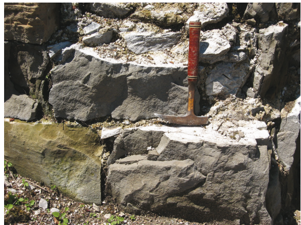
Fig. 9.14: Chiselled Oligocene sandstone blocks found in the foundation of the inner curtain wall. Such blocks were not found in the tower. While easy to chisel, this type of sandstone is prone to weathering. The two pedestals in the courtyard are made from the same sandstone.
