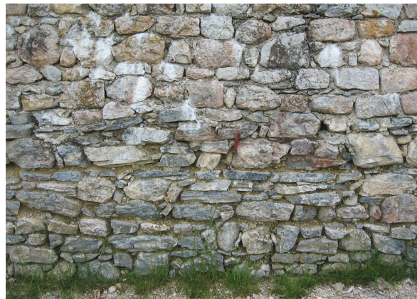
Fig. 9.8: The original lower and the reconstructed upper part of the tower wall.
