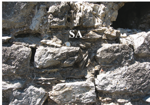
Fig. 9.11: Inner curtain wall. The stones are slightly better chiselled and provide a better fit. The blocks were chosen more carefully than in the tower and the construction was better. Fig. 9.8 shows a tufa block (L) between the quarry stones. Gaps in the wall were filled with smaller "schistose" limestone pieces (SA). View 2.
