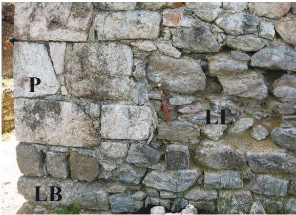
Fig. 9.7: Local quarry stones (LL) and limestone blocks from Povodje (P). The bottom two rows of the corner are original, made from smaller chiselled blocks of local black bedded limestone (LB). Larger chiselled blocks of Povodje limestone can be found higher up in the corner. The original wall was made entirely of local quarry stones, while the reconstructed one was made almost entirely of smaller, not so well chiselled blocks of Povodje limestone. Cement mortar was used between the Povodje limestone blocks, while the original stones were bound by limestone mortar with dolomite grains.
