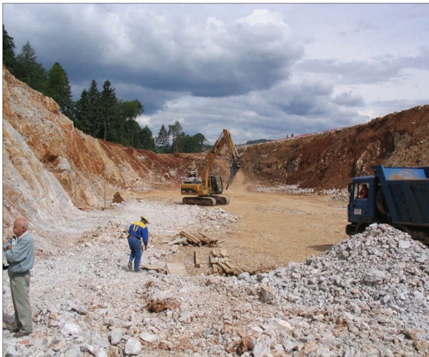
Figure 228 Construction of the highway north of Novo mesto has exposed profile of the laminated grey sediments, which were covered by red soil. The profile lies behind the drilling machine in the middle of the photo.
