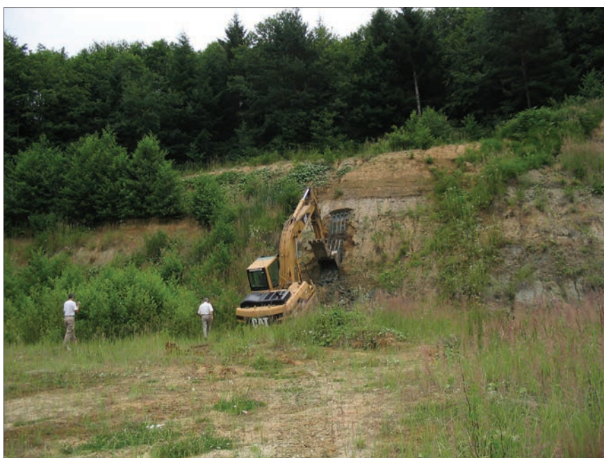
Figure 268 Excavation of the site, Velenje.
