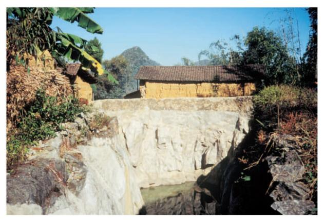
Fig. 2.10.13. Water reservoir by the village of Miandze, Xichou. The fissures widened by corrosion and filled with loam were used, this is indicated by the subcutaneous forms on the wall. (Photo A. Mihevc)
