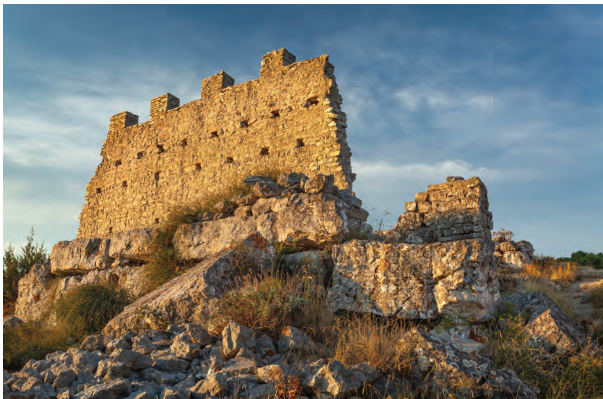
Sl. 12.14: Gradina, Žirje. V celoti ohranjen del obrambnega zidu s cinami na vrhu. Fig. 12.14: Completely preserved part of defence walls with merlons at the top.
