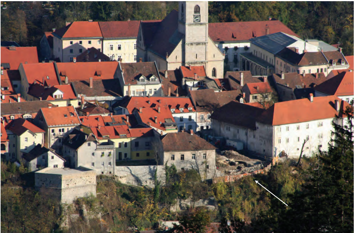
Sl. 12.8: Kranj. Pogled s severozahoda na del poznoantičnega obzidja s stolpom. Fig. 12.8: View from the north-west to a part of the late antique defence walls with a tower.
