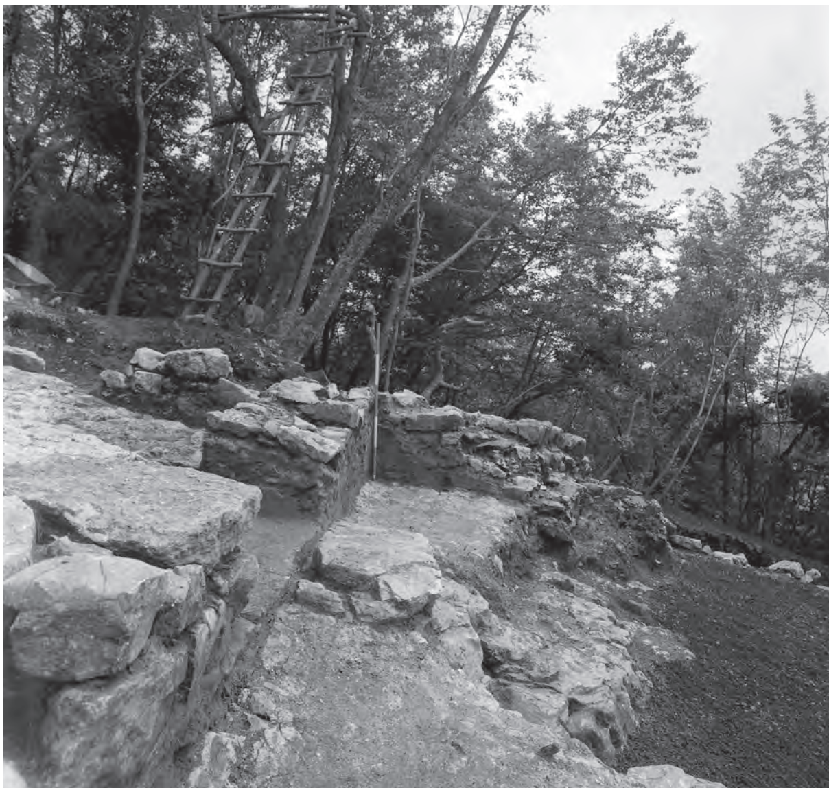
Sl. 2.30: Cerkev. Zid 1 s prehodom iz ladje v stranski prostor in stopnico pred prehodom. Pogled proti vzhodu. Fig. 2.30: The church. Wall 1 with the passage from the nave into the annex and the step in front of the passage. View towards the east.
