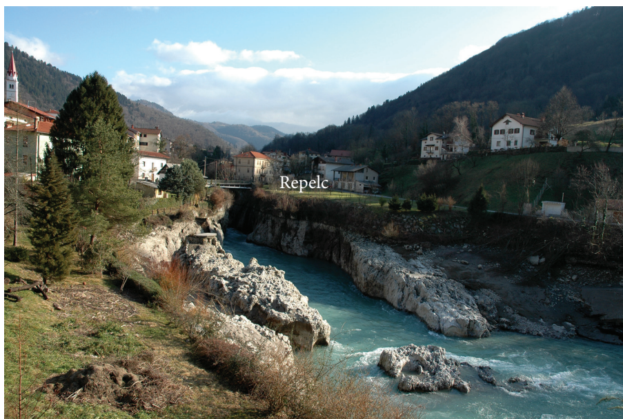
Sl. 20: Most na Soči. Repelc in korita Idrijce ob izpraznitvi jezera januarja 2018; pogled z zahoda. Fig. 20: Most na Soči. Repelc and the bed of the Idrijca after emptying the hydro dam in January 2018; view from the west.
