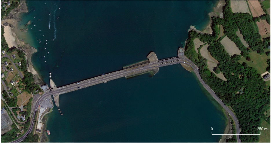
Figure 3: An aerial image of the Rance Tidal Power Station located in the Rance River estuary in France. Image captured from Google Earth.
