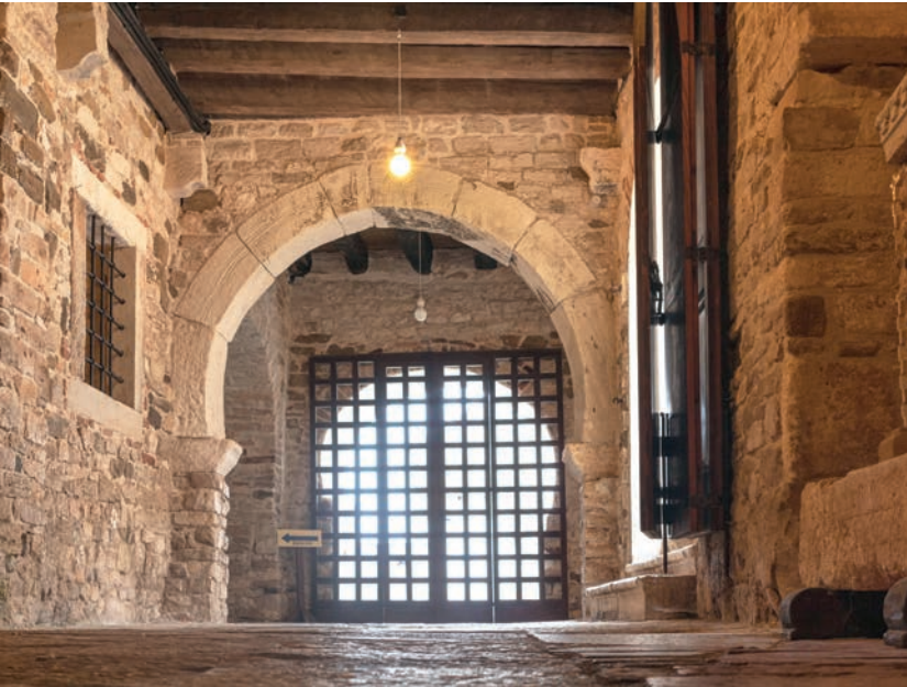
Fig. 2.255: Parentium. Ground floor rooms in the episcopium (2010).
