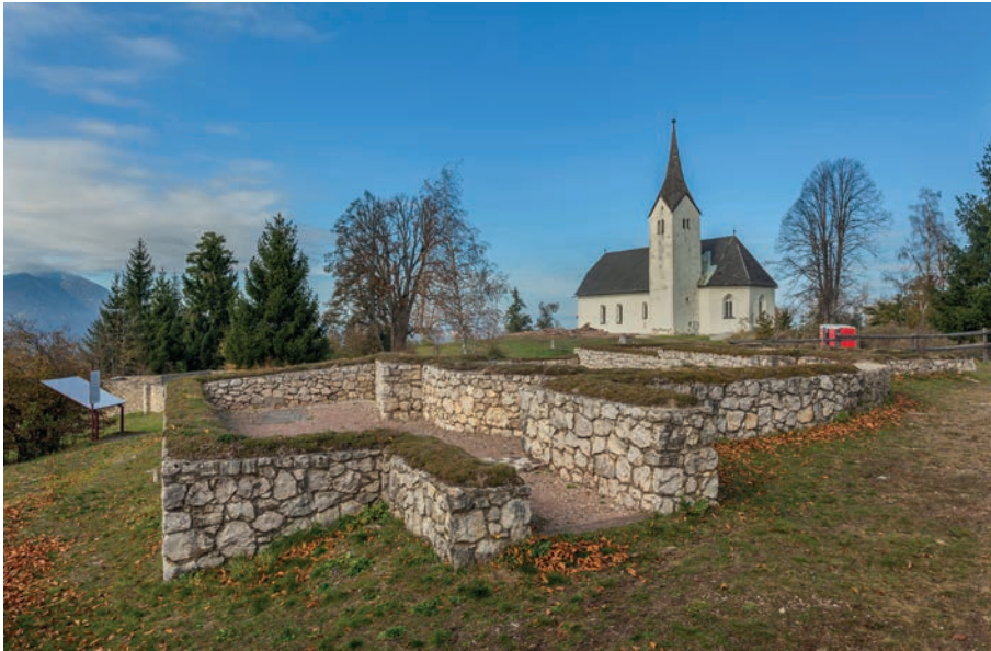
Fig. 3.311: Hemmaberg above Globasnitz. Remains of the earliest church at the top of the settlement plateau (2014).
