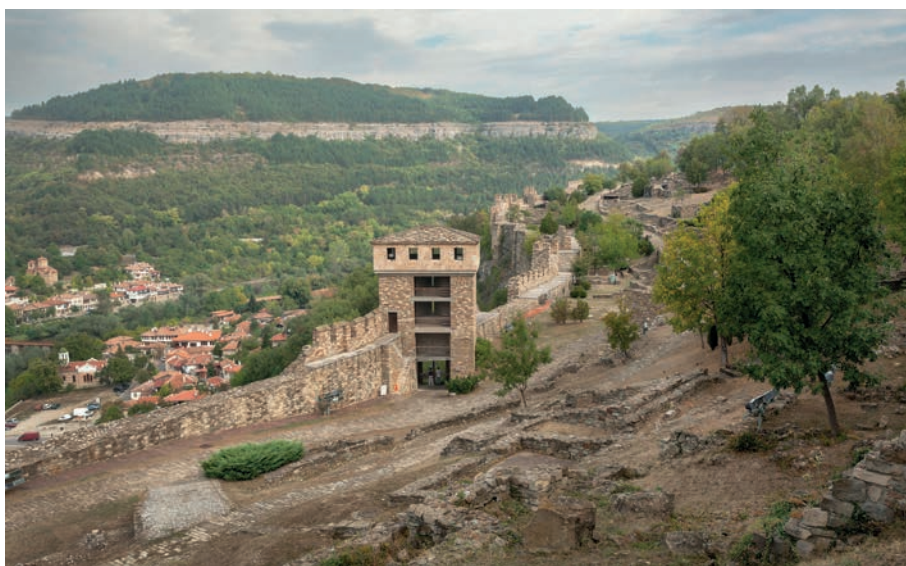
Fig. 2.204: Carevec. Walls and ruins of the buildings on the western side of the city (2012).
