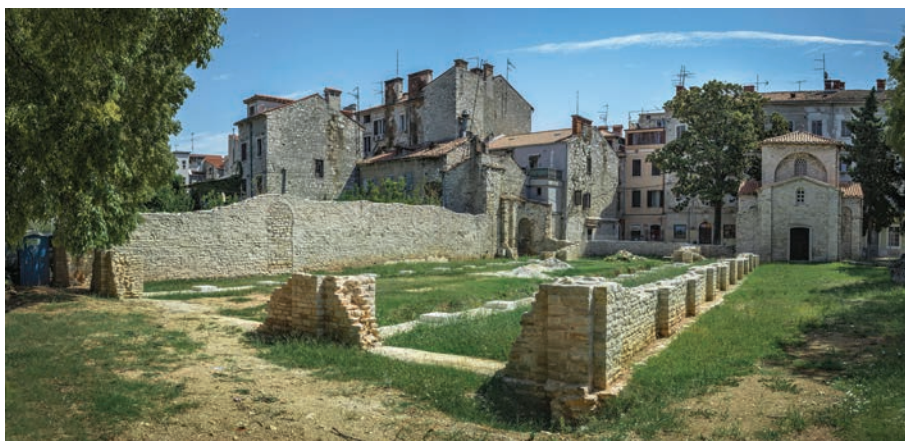
Fig. 2.52: Pola. Remains of Early Christian church of Maria Formosa with a fully preserved chapel (2014).
