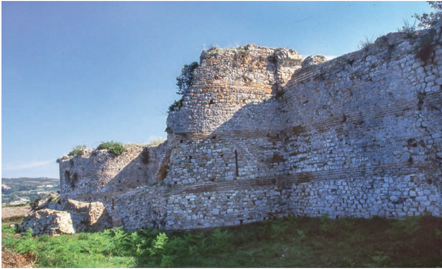
Fig. 2.259: Nicopolis in Epirus. Late Antique walls with towers (2002).
