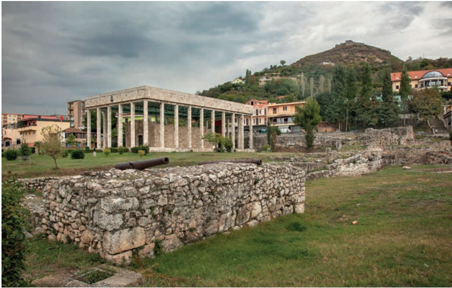
Fig. 2.101: Lissus. Remains of lower part of the city from the south-west with the acropolis at the background (2009).
