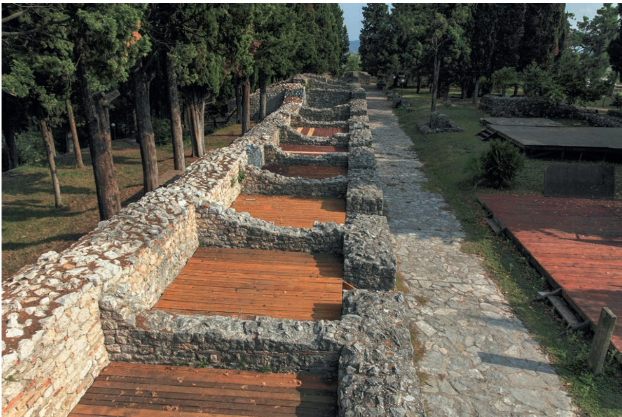
Fig. 3.193: Mogorjelo. Walls with residential buildings (2009).
