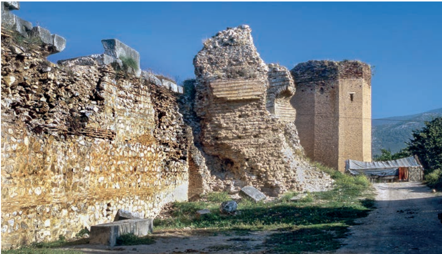
Fig. 5.35: Nicaea. Thick city walls from the early 4 th century (2003).
