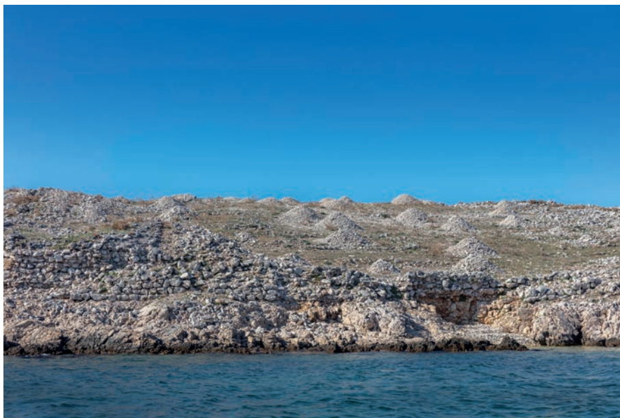
Fig. 3.152: Veliki Sikavac. Impressive defensive walls and the remains of the buildings on the eastern side of the fort (2016).
