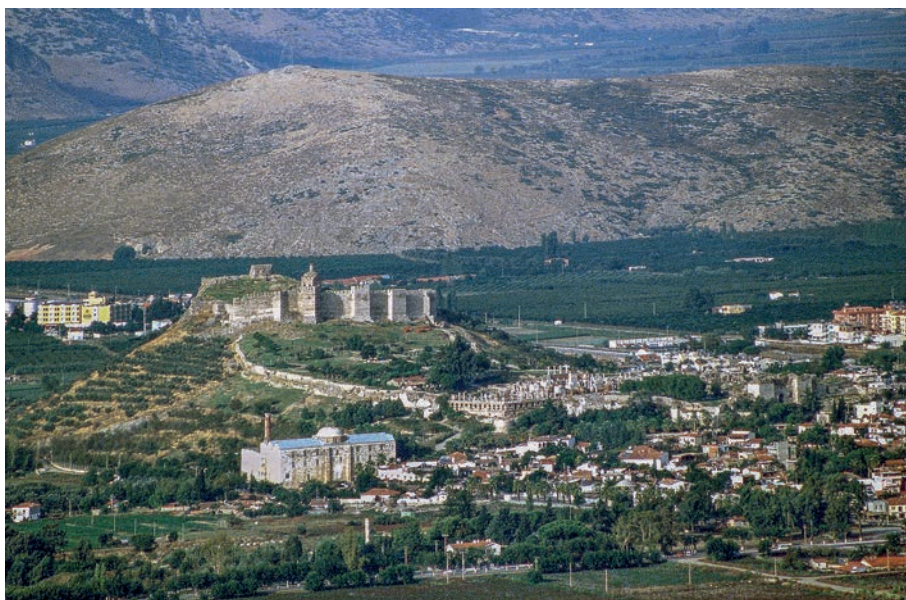
Fig. 5.29: Ephesus. A large pilgrimage centre formed in the 6 th century next to the church of St John (2002).
