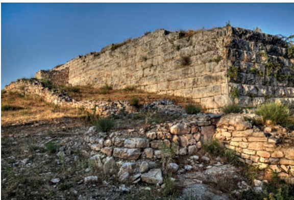
Fig. 2.58: Asseria. South-western corner of city walls with a tower and a proteichisma (2004).
