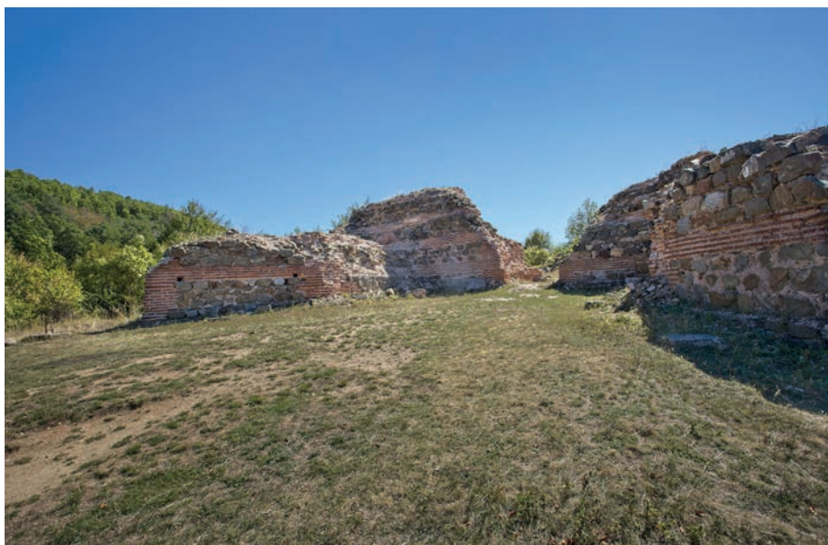
Fig. 3.247: Markova Mehana. Well-protected entrance (2012).
