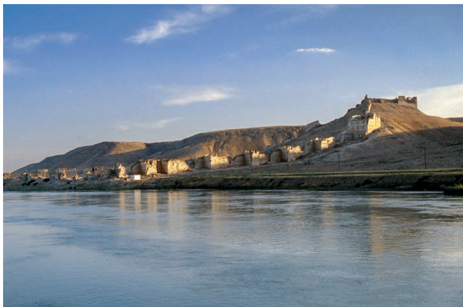
Fig. 5.39: Zenobia. Heavily fortified Early Byzantine city on the slope above the River Euphrates (2004).
