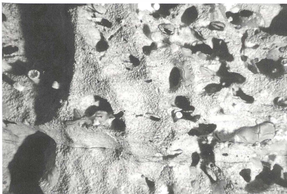
Fig. 6. Part of the cave wall with pronounced bivalve corrosion located between sections B-B' and C-C'.
