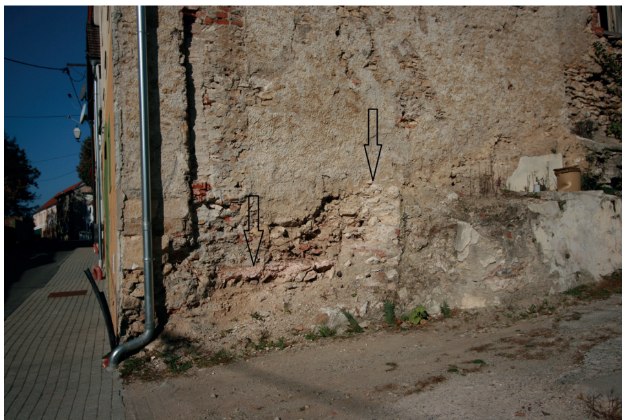
Fig 4: Varaždinske Toplice: Braće Radić Street, eastern wall of the house at number 5 with remains of the Roman wall and plastered floors. (Photo: D. Kušan Špalj)
