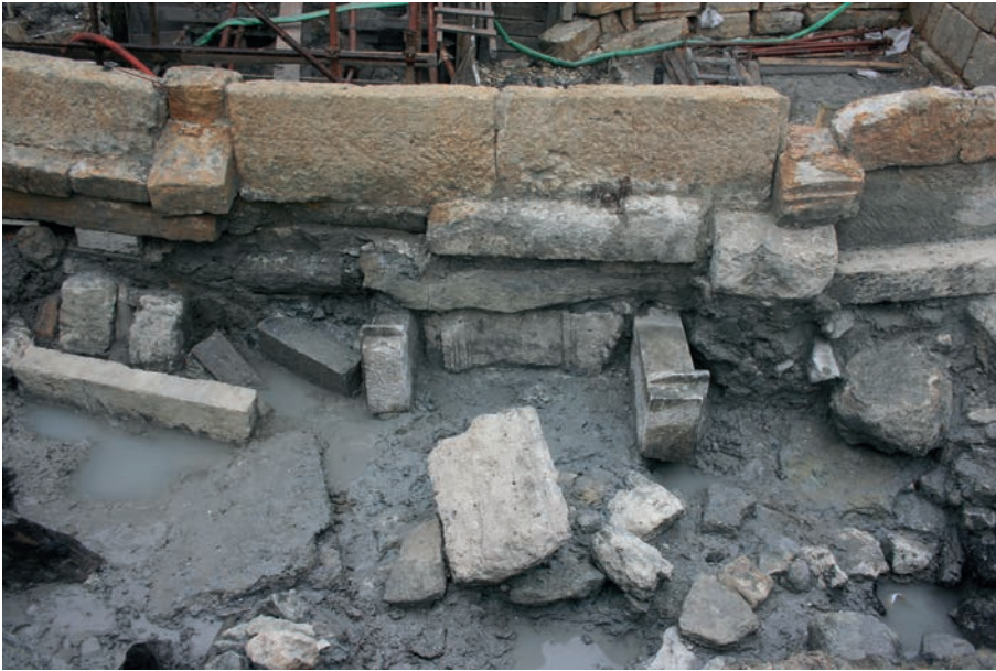
Fig. 18: Varaždinske Toplice, excavations in 2012. View to the back side of the southern wall of the spring reservoir. (Photo: D. Kušan Špalj)
