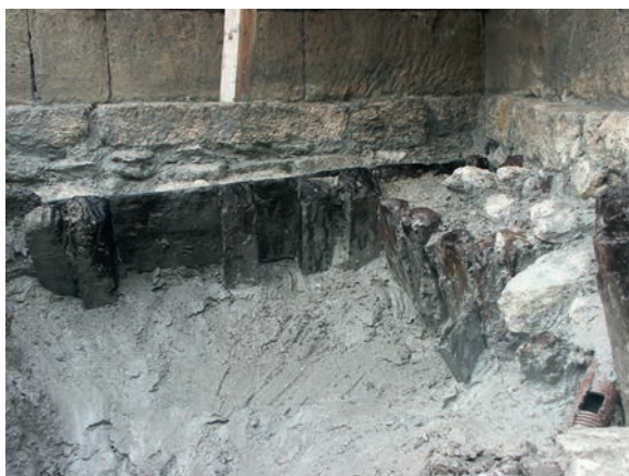
Fig. 8: Varaždinske Toplice, excavation in 2011. The piling system (2nd century) in northwest corner of the spring reservoir, view to the west. (Photo: D. Nemeth-Ehrlich)
