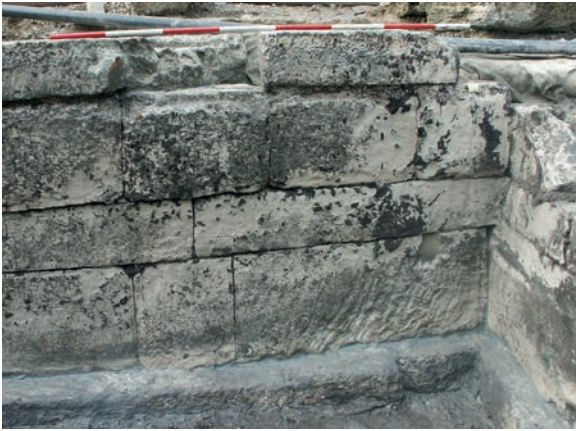
Fig. 9: Varaždinske Toplice. Western wall, northwest corner of the spring reservoir (2nd century). (Photo: D. Nemeth-Ehrlich)
