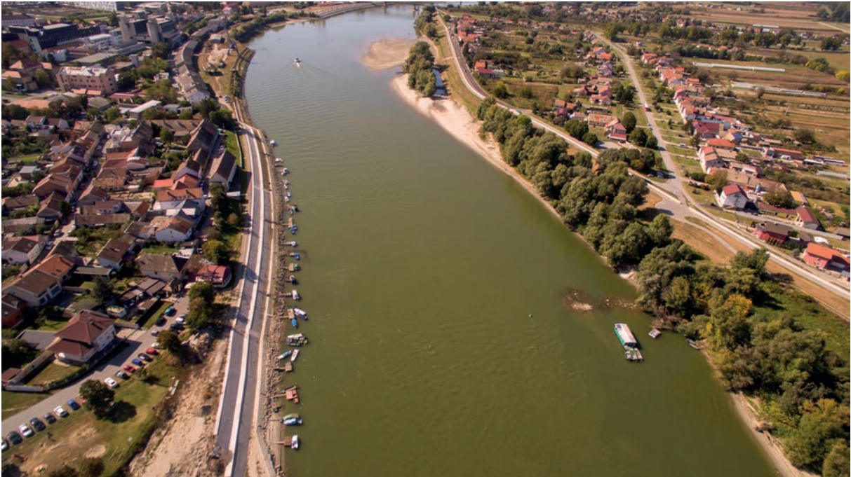
Fig. 9: Aerial photo of the Roman bridge in Mursa. View towards west.
