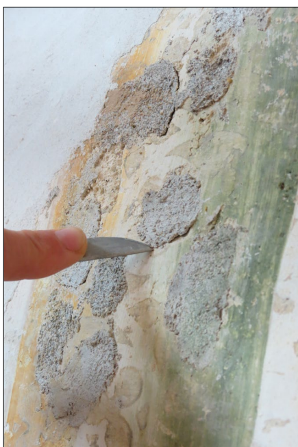
23.–24. Removing Stern's infillings and in-paintings which covered the Gothic painting. They were removed for technical and aesthetic reasons (© IPCHS, RC, photos: Anita Klančar Kavčič, 2014, 2006)
