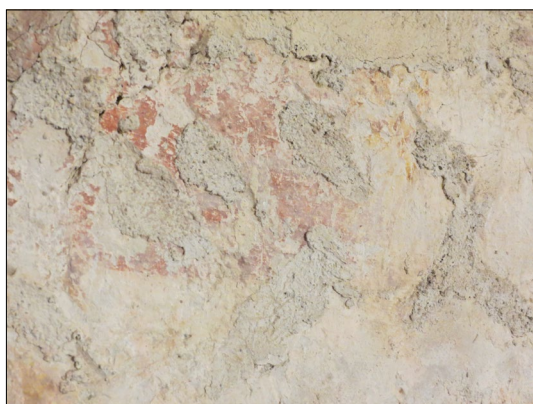
9.–10. Sternen filled losses in the plaster with lime mortar, taking no particular care to seal off the edges of the fillings, and so the rough surface of the fillings differs from the original surrounding plaster. He left some fillings uncoloured (left), while overpainting others (© IPCHS, RC, photos: Anita Klančar Kavčič, 2017)
