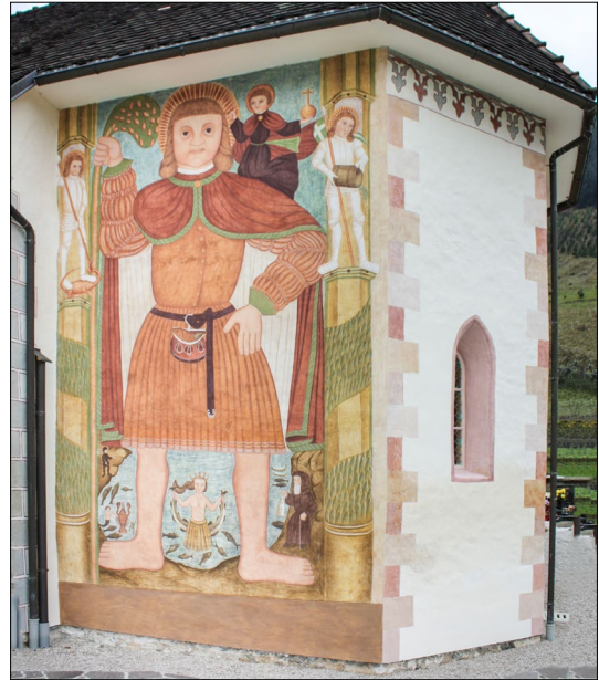
30. Exterior of the chancel after a copy was made of the monumental painting of St Christopher and after the reconstruction of the Gothic windows (Photo: Vid Klančar, 2008)
