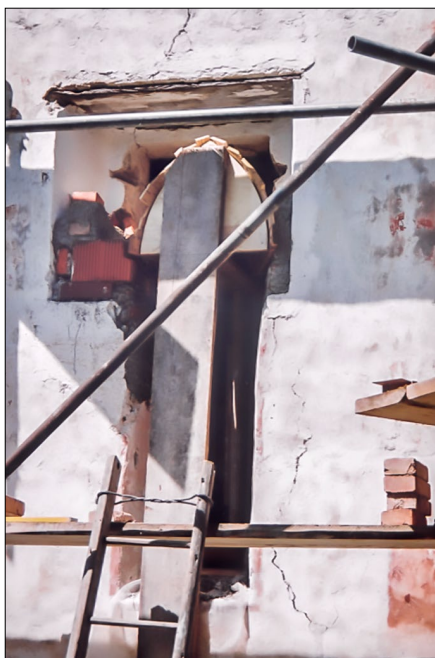
21.–22. In 2004, the reconstruction of the Gothic windows was carried out in the chancel. This intervention affected both the interior and exterior (Photos: Martina Lesar Kikelj)
