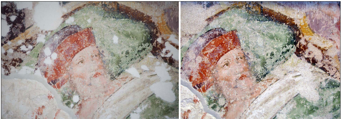
34. Restrained retouching, simulating painted plaster (intonaco) on the infillings and with colour glazes ( abbassamento di tono ) on abrasions represents the conservation approach in the Church of the Assumption in Bled (Photos: Jelka Kuret, 2016)
