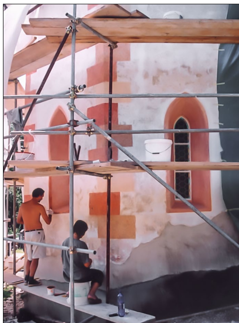
21.–22. In 2004, the reconstruction of the Gothic windows was carried out in the chancel. This intervention affected both the interior and exterior (Photos: Martina Lesar Kikelj)
