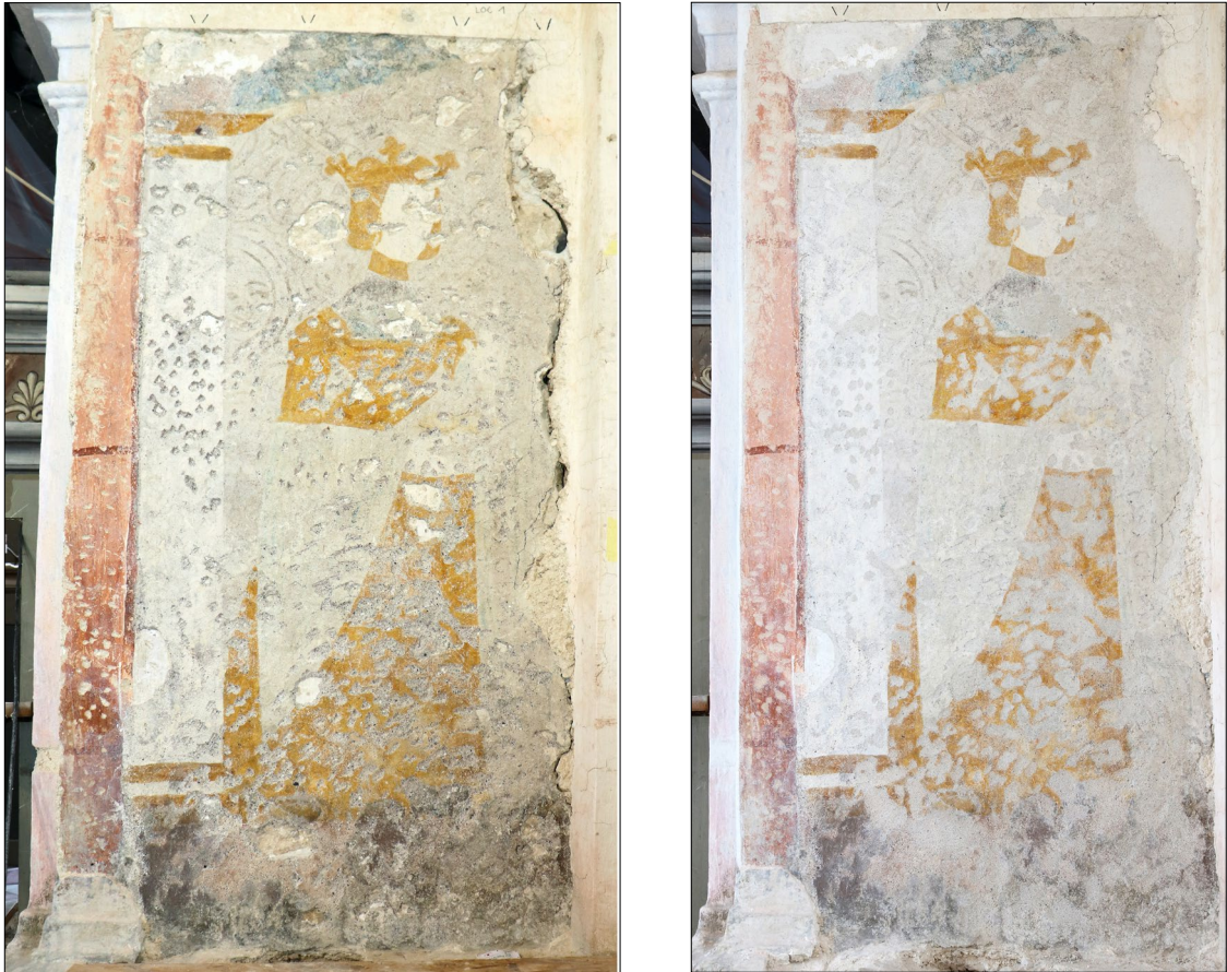
36. Šentjošt nad Horjulom, church of St Judoc. The prominent damage and cracks are infilled with mortar, which contains different colour aggregates and is thus already tonally adapted to the tone of the intonaco. In this way, the image is assembled into a whole without retouching with colour (Photo before the intervention: Marija Eva Fras, 2020; photo after the intervention: Anita Kavčič Klančar, 2021)
