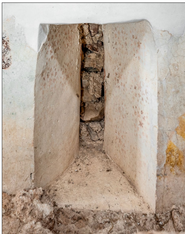
21. Turjak Castle, Romanesque window in the southern wall of the former Romanesque chapel (© ZRC SAZU, UIFS, photo: Andrej Furlan)
