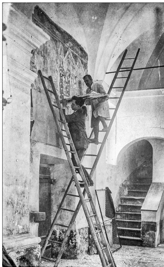
5. Matej Sternen and France Stele during the detachment of the younger layer in the nave in 1925 (© Ministry of Culture of the Republic of Slovenia, Heritage Information and Documentation Centre, Ljubljana (INDOC Centre), photolibrary)
