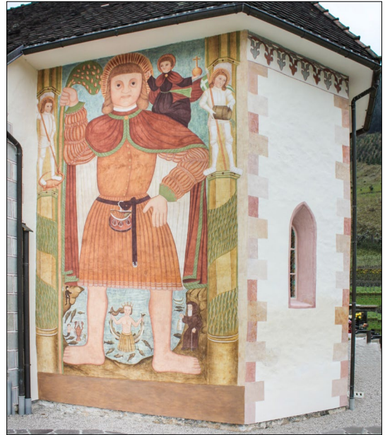
30. Exterior of the chancel after a copy was made of the monumental painting of St Christopher and after the reconstruction of the Gothic windows (Photo: Vid Klančar, 2008)
