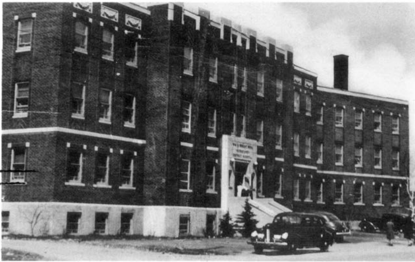
Kirkland Lake and District Hospital, Kirkland Lake, Ont.—29.
