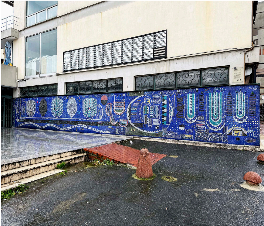
Figure 14. Bedri Rahmi Eyüboğlu's mosaic mural integrated into the façade of a shop in Block 2. Photo: İnan Kenan Olgar, 2025.
