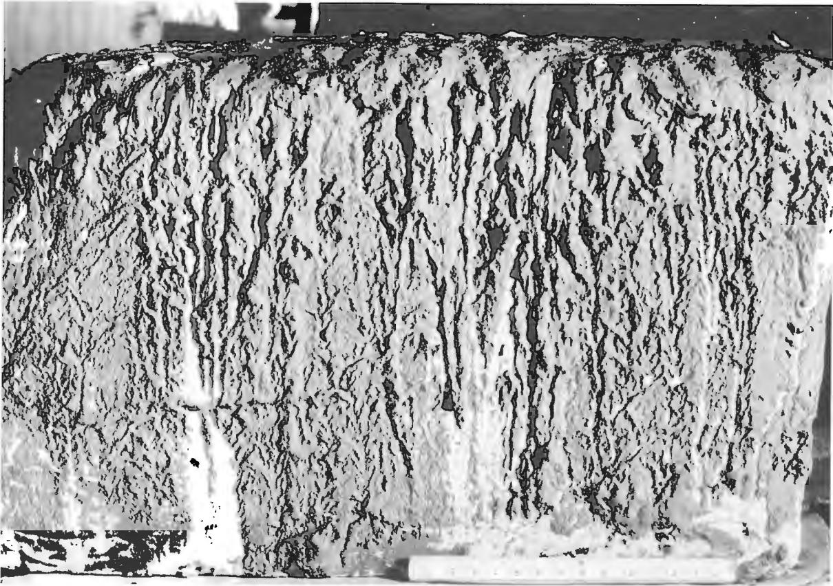
2.4.15 Channels on vertical wall of plaster block (scale = 15 cm)
