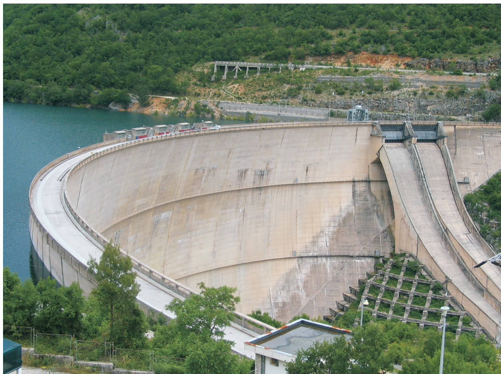
Fig. 38: Grančarevo dam in the upper part of Trebišnjica valley. Behind the dam, Bileća lake with storage capacity of 1,28 billion m 3 (Milanović 2004) was formed and flooded spring of Trebišnjica (photo: A. Mihevc).
