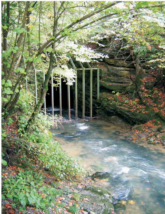
Fig. 36: During Austro-Hungarian Empire and Yugoslavia kingdom surface streams were regulated, ponors were widened and screens were installed in front of them to hold back deposits, all in order to shorten the flood time in karst poljes. Example from Šica ponor at Radensko polje (Račna polje; Slovenia; photo: M. Prelovšek).
