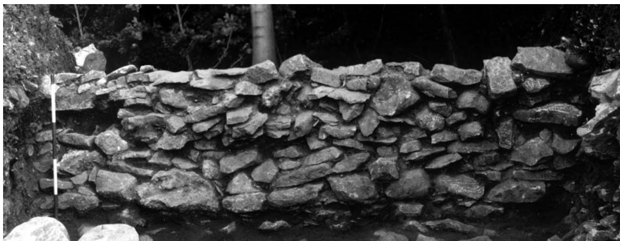
Fig. 50: Veliki Vinji vrh near Bela Cerkev. Wall III.
