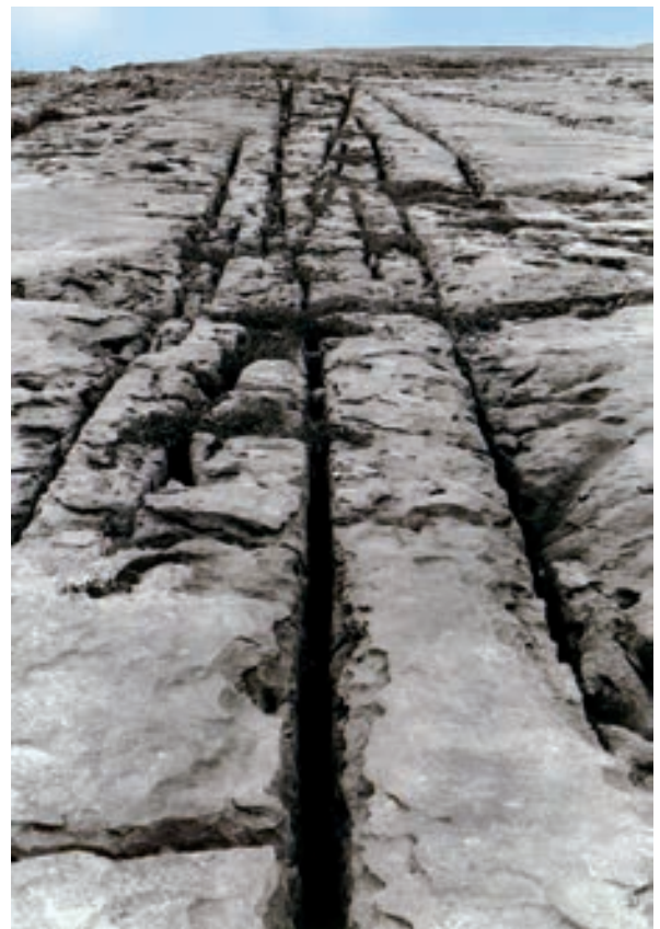
Figure 9: Burren, Ireland. Pavement showing differences between strength of two joint sets.
