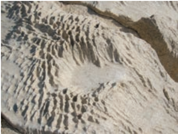
Figure 2: Rillenkarren features developing on gypsum blocks, after one century of exposure to rainfall, at the Minoan Knossos Palace (Crete, Greece). Width of view is 15 cm.
