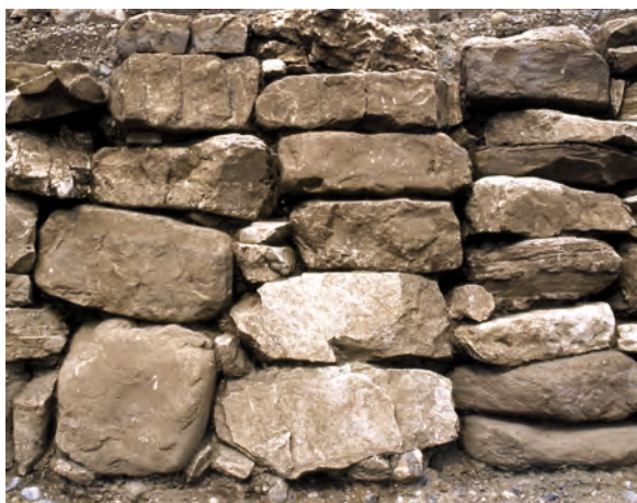
Sl. 153: Hiša 22. Gradbena faza 1, drenažni zid; pogled z juga. Fig. 153: House 22. Construction Phase 1, drainage wall; view from the south.
