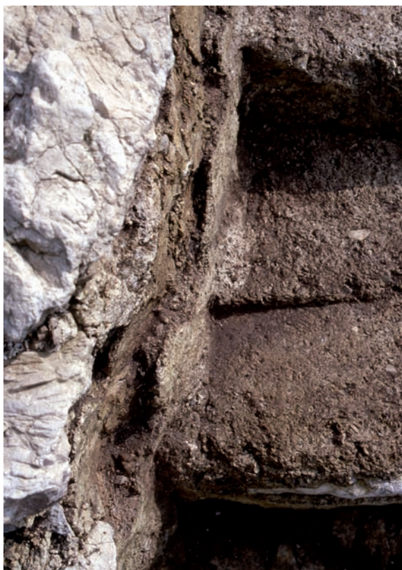
Sl. 2.66: Stopnici v ladji osrednje cerkve. Fig. 2.66: Stairs in the nave of the main church.
