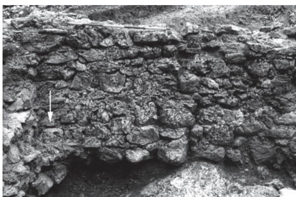
Sl. 2.18: Stavba 1, stik zidov 3 in 4. Iz malte oblikovana polička v kotu. Fig. 2.18: Building 1, contact between walls 3 and 4. The mortar shelf in the corner.
